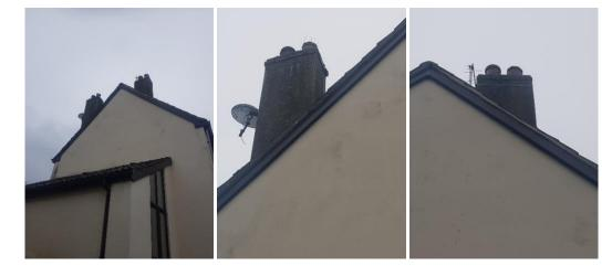
The chimneys appear upright with no signs of any significant bulging, twist or distortion.
