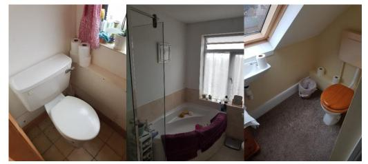
There were no extractor fans fitted to the bathrooms. Extractor fans are important to be used when the bathroom is in use so that condensation and water vapour is removed. Excess build-up of condensation and water vapour can lead to dampness and mould. The extractor fan will help to stop this problem from occurring.
