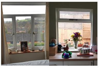
Window openings are square to the eye with no signs of any significant movement or distortion noted. Routine maintenance is advised to keep the windows functioning adequately. Hinges and locking mechanisms will need to be regularly lubricated in order to prolong their lifespan and efficacy.
