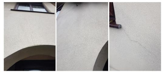
The render to the exterior wall of the kitchen is badly weathered/worn and is in need of decoration to prevent further damage and water ingress.
