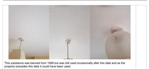
Asbestos is quite safe unless split or cracked when it becomes dangerous. It should not be tampered with in any way. If it is required to work on the ceiling – a specialist firm must be employed to carry this out.
